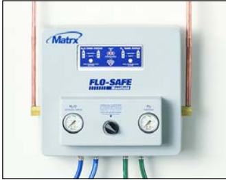
Flo-Safe Manifold (for built-in central gas supply)
